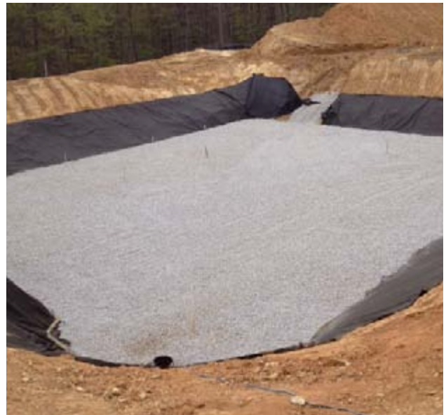
Line trench walls, not trench bottom, with StormChamber® filter fabric.
