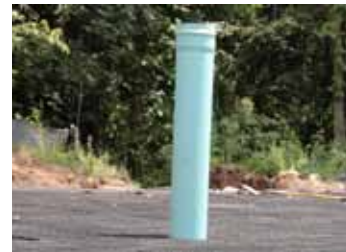
Fig. 16 Installed maintenance port
