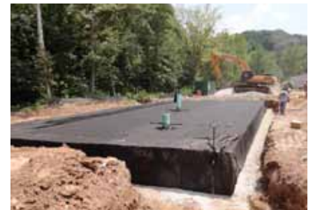
Fig. 22 "Walk" the geotextile into the corner to eliminate air gaps.
