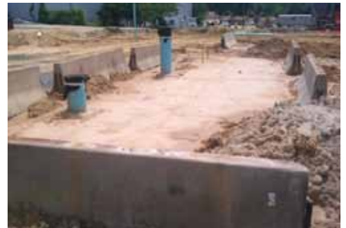
Fig. 28 Secured R-Tank HD installation using Jersey Barriers.
