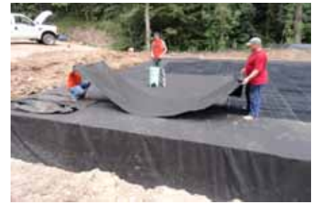
Fig. 20 Encapsulate R-Tanks HD with geotextile.
