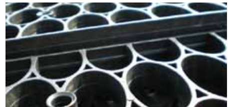
Fig. 9 Minor variations (less than width of top plate) in tank height are acceptable.
