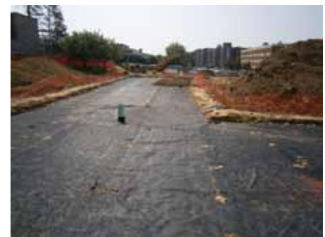
Fig. 25 Overlap Geogrid 18" or as required by plans.
