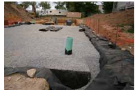
Fig. 24 Use an LGP dozer to push backfill over R-Tank HD units.
