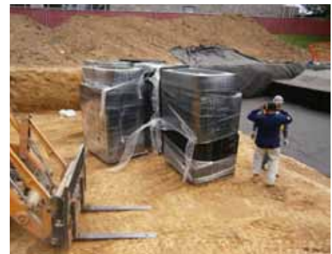
Fig. 3 Installation can be sped up by either assembling the tanks in the excavation or placing the pre-assembled tanks in the excavation.
