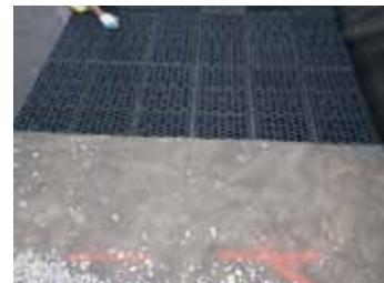
Fig. 18 Maintain 12" overlap on textile.
