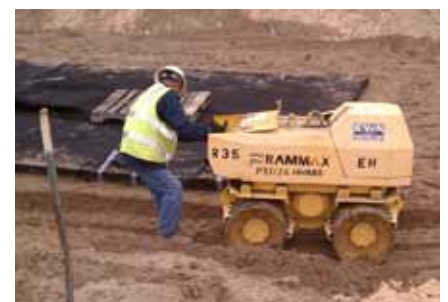
Fig. 23 Vibratory compaction of side backfill is ALWAYS REQUIRED, regardless of what backfill material is used.
