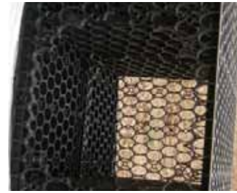
Fig. 15 If after adjusting the internal plates, the pipe will not fit, the top plate can be cut off-center and one of the internal plates can be removed.
