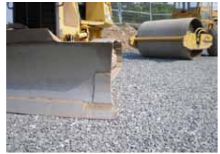
Fig. 4 Base must be smooth to ensure units fit together without gaps.
