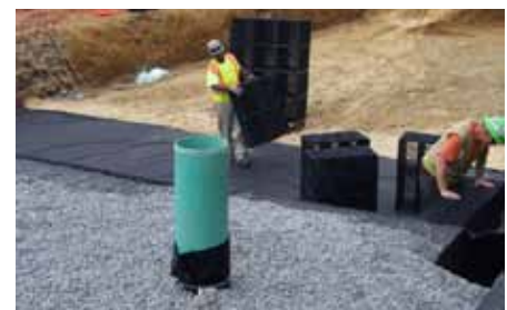
Fig. 11 Installed Inspection Port
