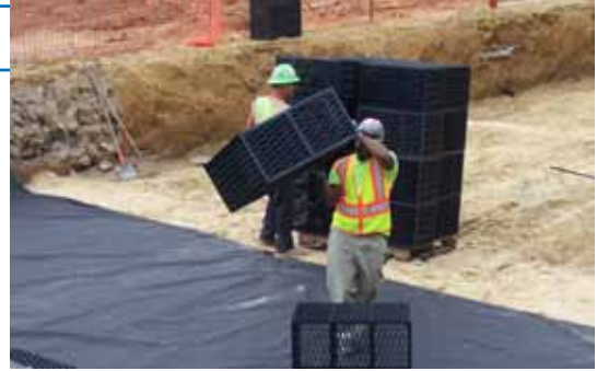
Most contractors find installing an R-Tank ® system surprisingly easy.
