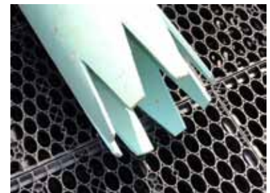
Fig. 14 Cut 8" notches into the bottom of Maintenance Port.
