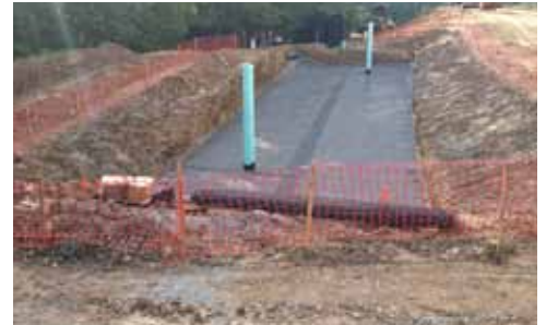
Fig. 27 Secure the installation with temporary fencing.
