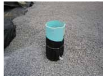
Fig. 17 Install port into R-Tank HD .
