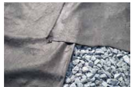
Fig. 6 Reduced overlaps don't create significant savings and can create delays.
