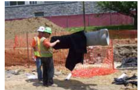
Fig. 21 Seal the pipe boot with the included band clamps and duct tape.
