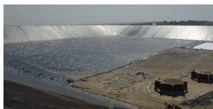
[Hydro Power Plant Application]
