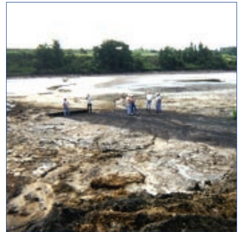
Mead paper mill landfill closure, MS 330 geogrid for fly ash stabilization. Grand Prairie, TX, sludge landfill capping, MS 550 geogrid for stabilization.
