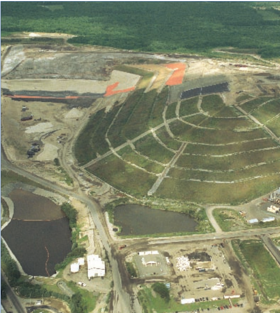
Central landfill final cover, Tenflow for surface water drainage, Rhode Island.
