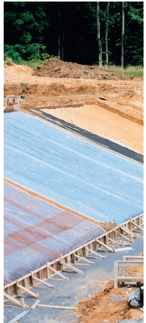
Irwin Creek flow equalization facilities, Tendrain for subsurface drainage, North Carolina.
