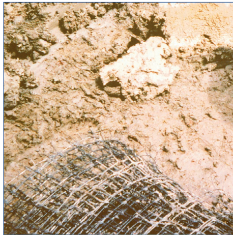
Mead paper mill landfill closure, MS 330 geogrid for fly ash stabilization. Grand Prairie, TX, sludge landfill capping, MS 550 geogrid for stabilization.
