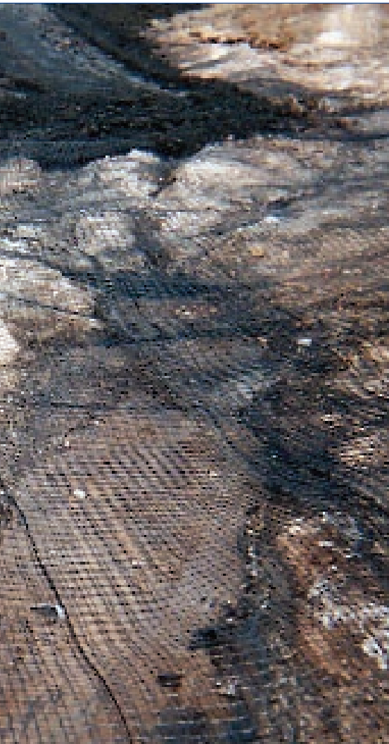
Mead paper mill landfill closure, MS 330 geogrid for fly ash stabilization. Grand Prairie, TX, sludge landfill capping, MS 550 geogrid for stabilization.
